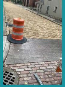
Hessler Street, Cleveland's last remaining wood brick roadway, underwent a major restoration. Originally replaced in the 1980s, the wooden bricks had since deteriorated, succumbed to rot, potholes, shifting bricks, and poor drainage, with only patchwork repairs over time. In a two-month, \$700,000 effort, the street was meticulously reconstructed, brick by brick, using durable Black Locust wood blocks.
